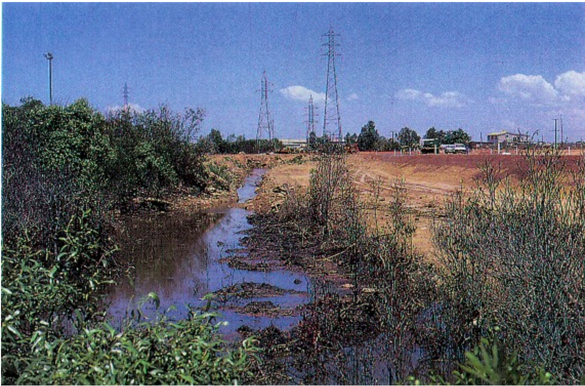
Plate 5 Pooling of stormwater through inadequate drainage creates mosquito breeding sites.
