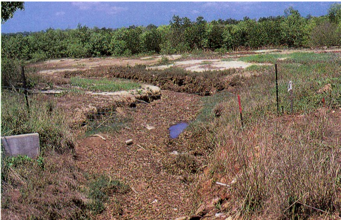
Plate 2 An artificial drain constructed without an outlet to the tidal zone will simply pond and stagnate – and breed mosquitoes.
